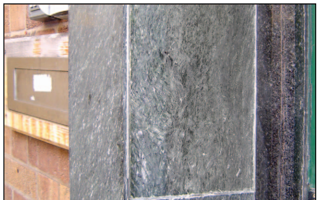
Figure 18. Phyllite cladding on Walkabout (92).
