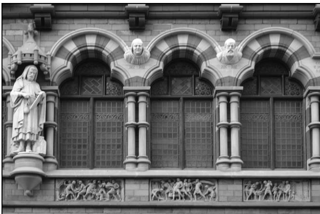
Figure 11. Architectural detail by Watson Fothergill (33).
