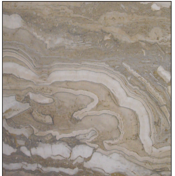
Figure 17. Travertine cladding on MacDonalds (83).
