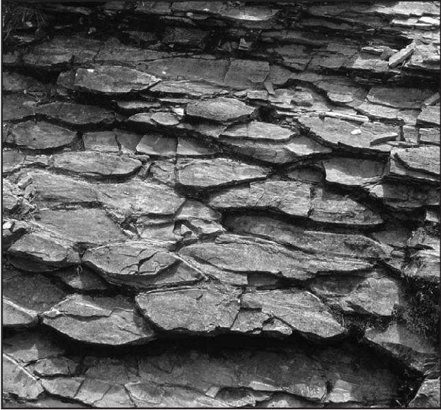
Figure 2. Basement jointing at Austwick Beck Head.
