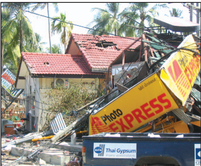
Figure 7. Concrete buildings survived in Phuket, Thailand, but the ground floors of frailer structures were washed out by the swirling tsunami waters (photo: Liz Price).
